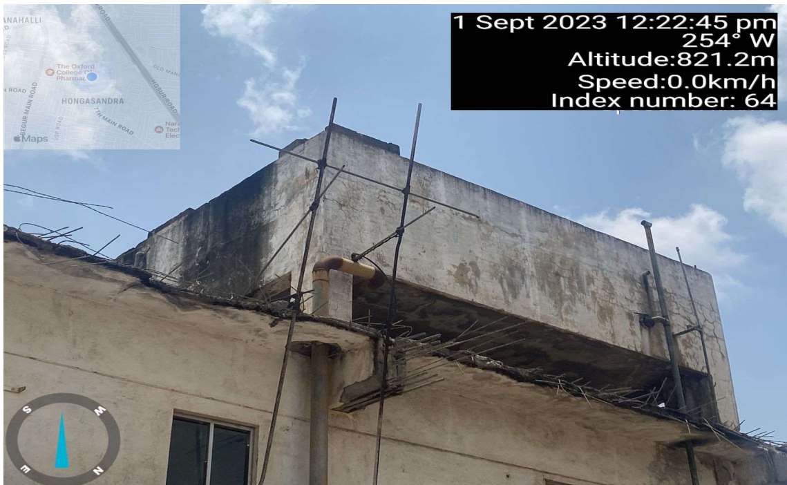
Construction of Tanks and Bunds - Overhead tank in the Girls Hostel
