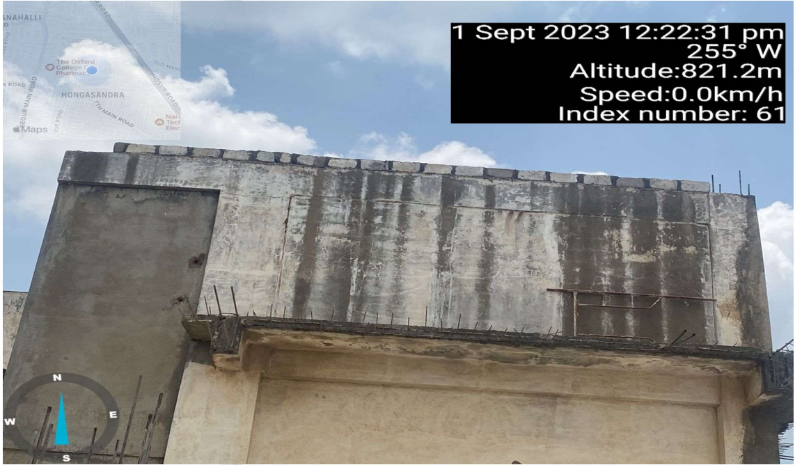
Construction of Tanks and Bunds Overhead tank in the College Building
